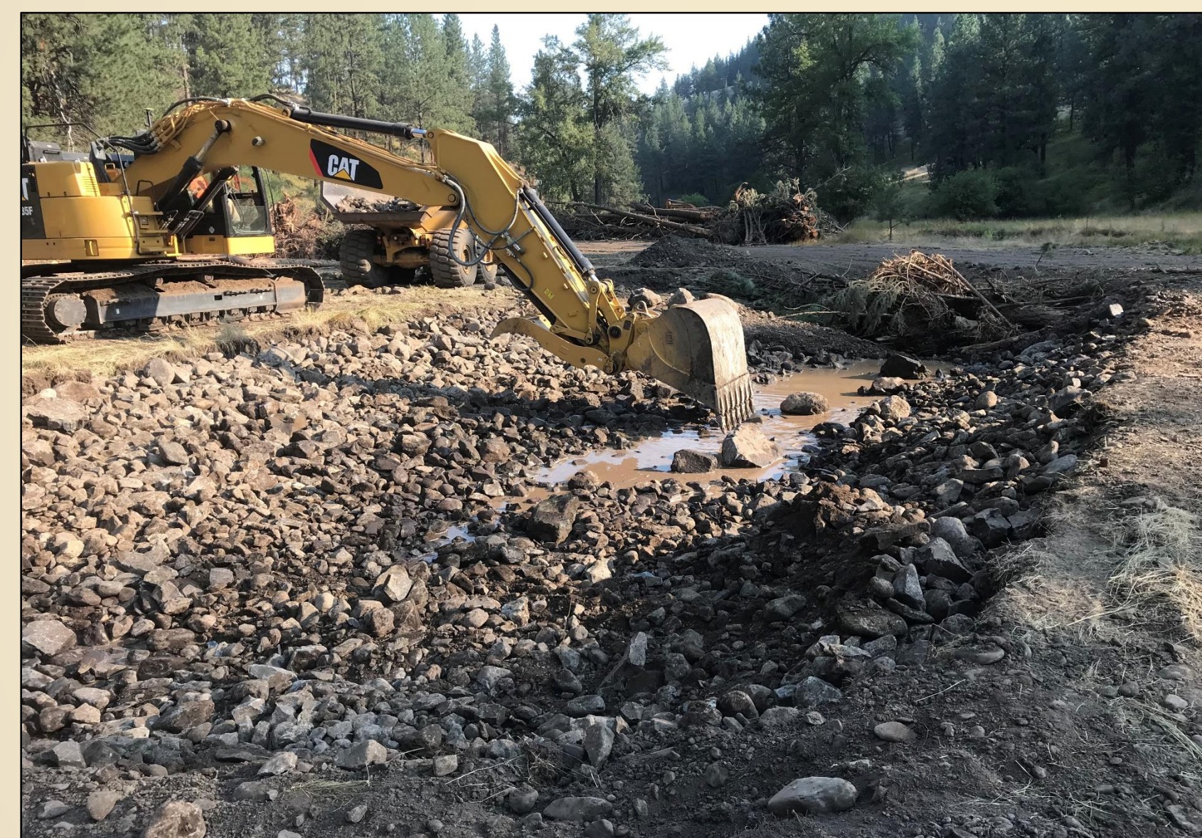
Rock Creek riffle construction, September 6, 2018 (looking upstream).
