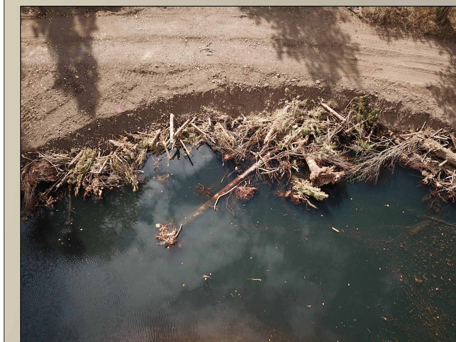
Completed large wood fish habitat structures on the Grande Ronde River.
