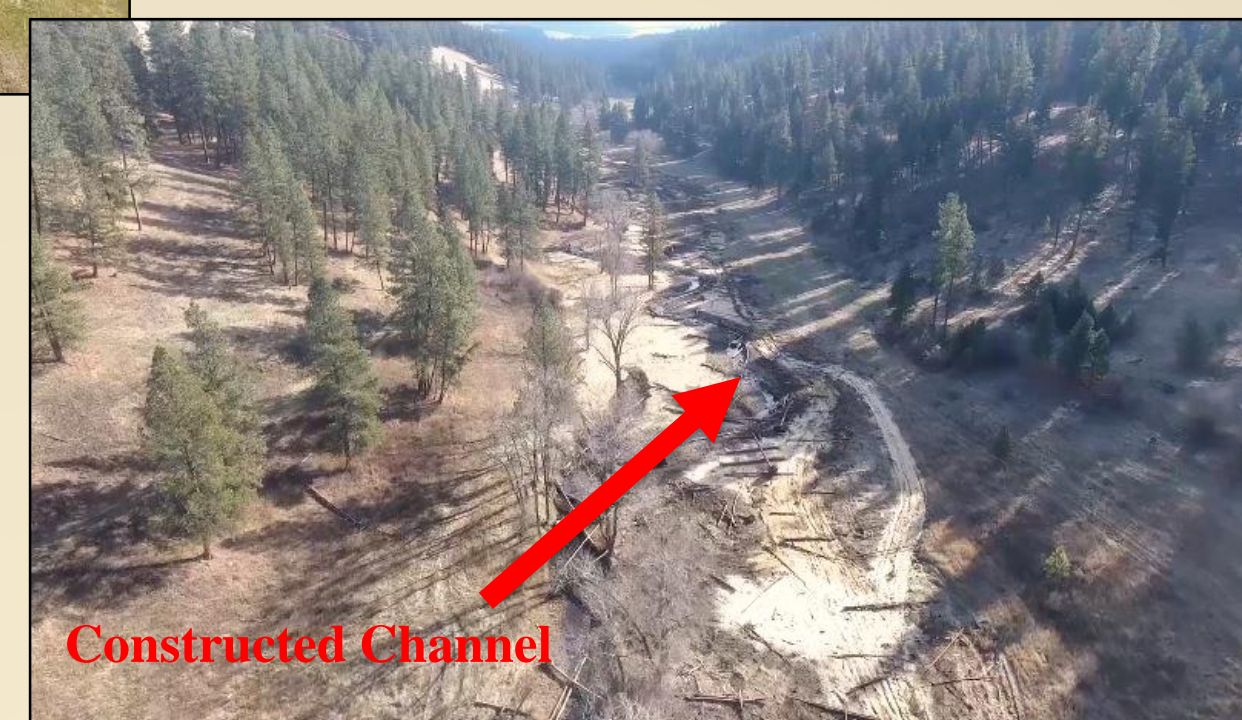
Rock Creek post-project photo November 20, 2018 (looking upstream).
